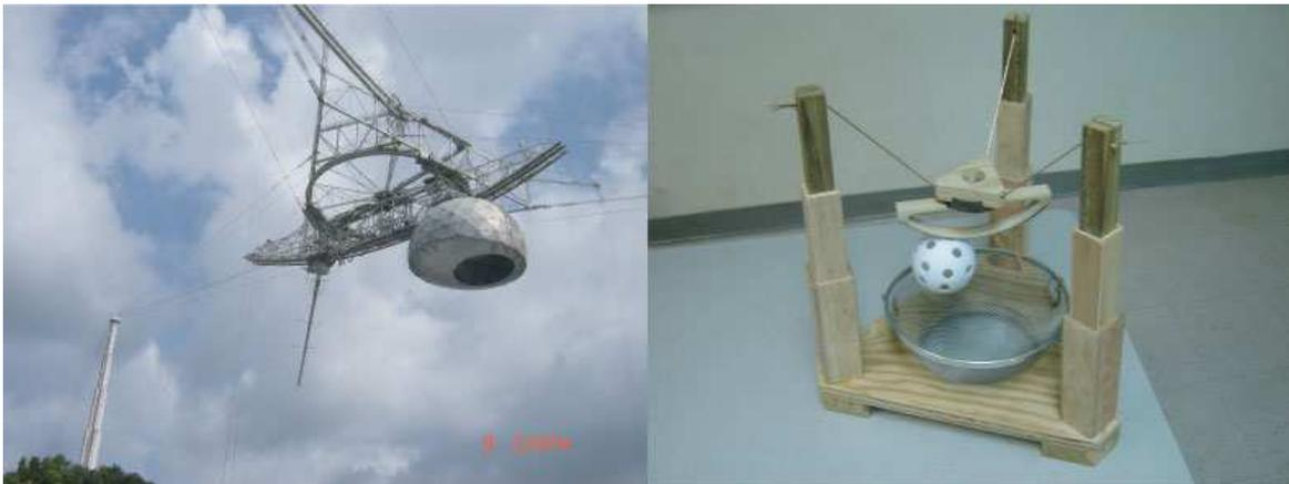
**Figure 4.** A view of the concrete tower, cables, triangular platform with circular track, azimuth arm with Gregorian dome, and carriage house (left), and the wooden model of the radio telescope (right).
