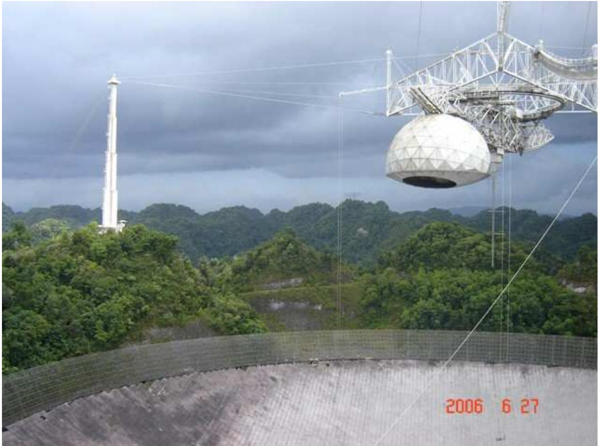
**Figure 1.** The main spherical dish of the Arecibo Observatory radio telescope (below), one of the concrete towers (left) that holds, by means of cables, the triangular platform (above) with the Gregorian dome and the 430MHz line feed suspended below it.
